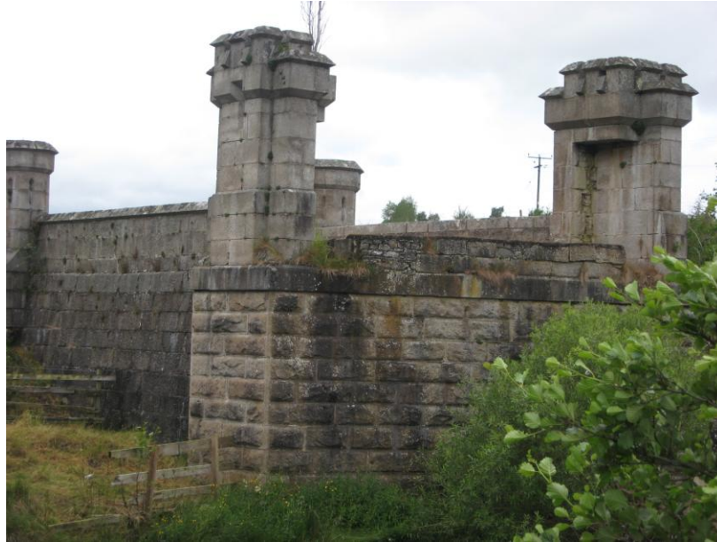
Figure 2 – photo of existing bridge
